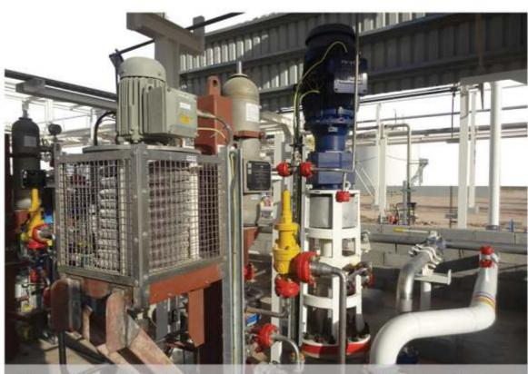
Closed Drain Vessel Pumping Oil & Water at Group Gathering Station
