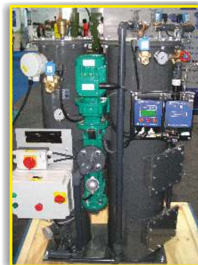
Roto Pump feeding oily water on OWS
