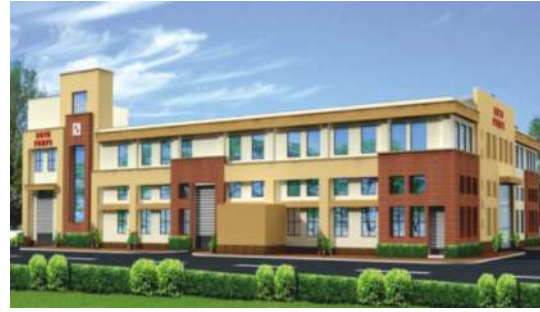
Roto Manufacturing Plant
